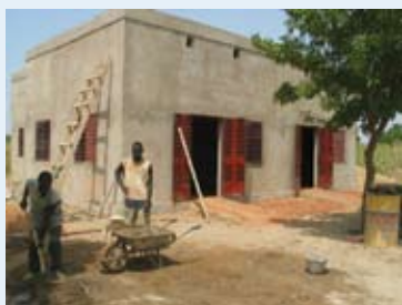
The new dental clinic being built
